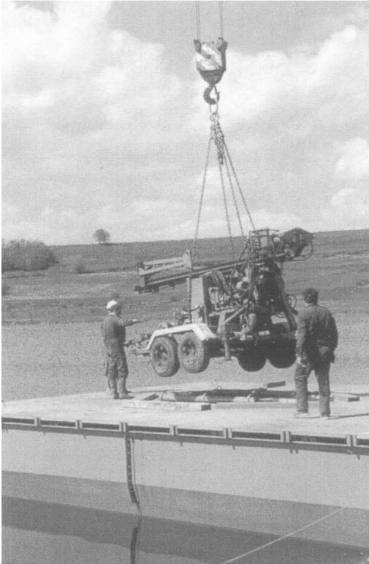
Figure 5. Sedidrill moved by a crane onto a platform on Lake St-Front, France (photo J.-L. de Beaulieu).
