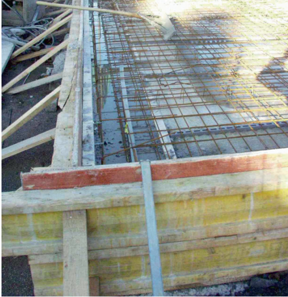
Fig. 27.8 Foundation earth electrode in construction
