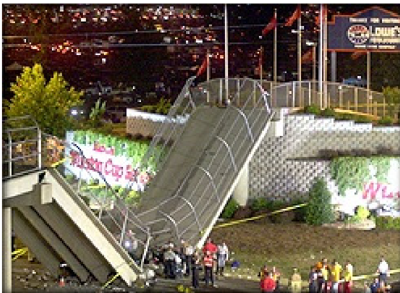
Figure 4.11: Example of collapse of a pedestrians bridge due to pitting corrosion of tendons, Concorde, USA 2000.
