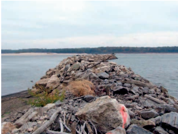
Figure 3 A dike constructed of rock riprap in the Mississippi River. These structures, although artificial, contribute greatly to stable substrate availability for invertebrate communities.
