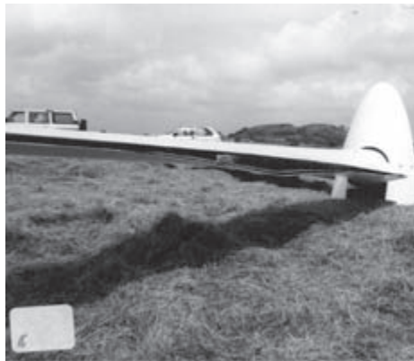
Figure 14.15 Blade ripped apart in the glued interface along the trailing edge by a lightning arc inside the blade (photo by the author)
