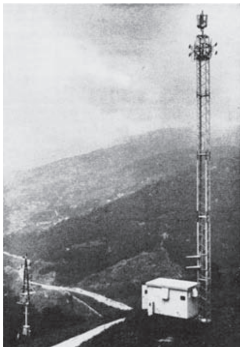
Figure 15.6 A typical low-power television and VHF/FM rebroadcasting station
