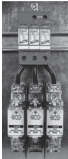
Figure 7.87 Application of DEHNguard surge arrester, DG TNC FM, U_c = 750 \text{ V}
