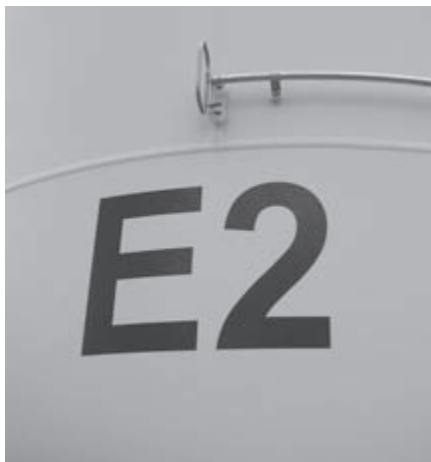
Figure 14.24 Lightning sensor antenna on wind turbine tower (photo by the author)
