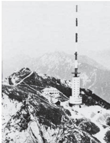
Figure 15.8 A typical large-scale television and VHF/FM broadcasting and radio relay station
