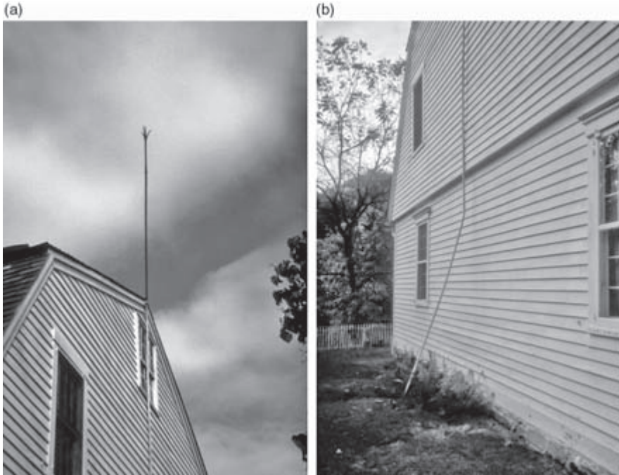
Figure 1.5 An eighteenth-century house with a lightning rod of Franklin's 1762 design. The thick, continuous rod can carry tens of kiloamperes of current to ground without harming the house or its foundation (photograph by the author).
