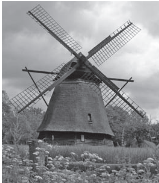
Figure 14.1 Windmill in the open air museum in Odense, Denmark. It is a wood construction thatched with straw (photo by the author).
