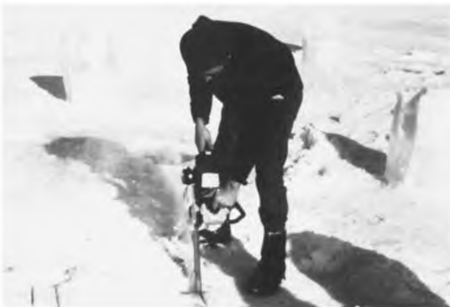
FIGURE 32. Hole cutting with a chain saw.
