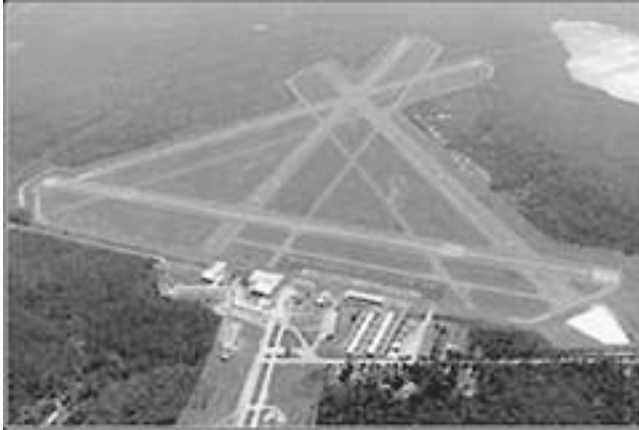
Figure 4-2. Flagler County Airport in Bunnell, Florida, has multiple crosswind runways to accommodate smaller aircraft in variable wind conditions. (Photo courtesy Se h Young)
