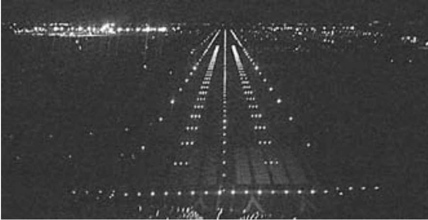
Figure 4-17. In-runway lighting at Daytona Beach International Airport. (Photo: J. Lukas k)
