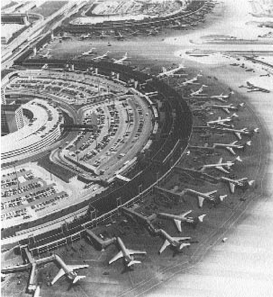
Figure 6-5. DFW Airport, whose terminal area employs a multiple-unit curvilinear terminal concept, now accommodates a large percentage of transfer passengers. (Photo courtesy FAA)
