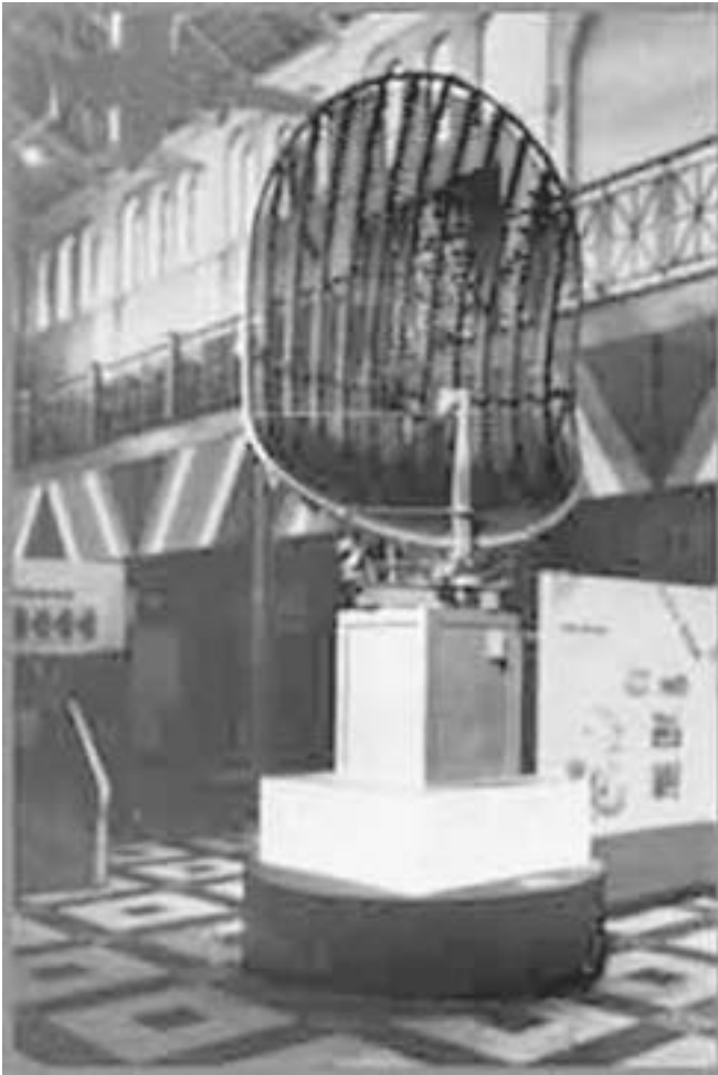
Figure 5-2. Early airport surveillance radar.
