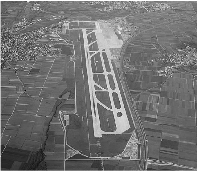
1.15 Airport expansion consists in providing new links in each part of the system. Stuttgart Airport, Germany. Architects: Von Gerkan, Marg & Partner.
