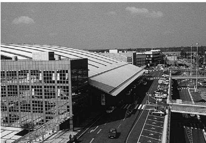
16.13 Hamburg Airport, Germany. Architects: Von Gerkan, Marg & Partner.
