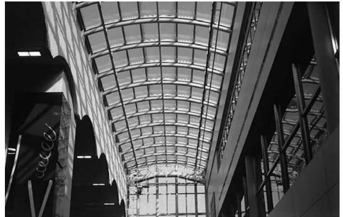
19.6 When Glasgow Airport was extended (right) a generous area of roof glazing was provided to create natural light in the centre of the terminal. The original terminal (left) was designed by Basil Spence in 1960.
