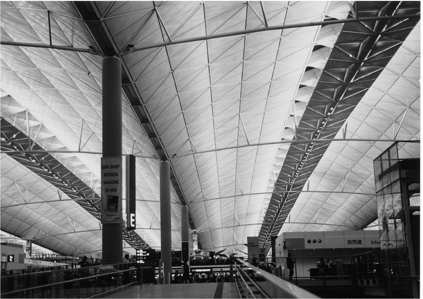
20.3 For the terminal designer light is a tactile material, which can be moulded and manipulated like any other. Light mixed with structure and interior space is the essence of the architectural experience. Hong Kong's airport at Chek Lap Kok. Architects: Foster and Partners.
