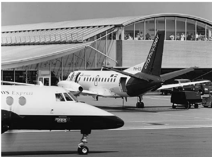
1.4 Even regional airports such as Southampton enjoy the benefit of commuter and international travellers. Southampton Airport, UK. Architects: Manser Associates.
