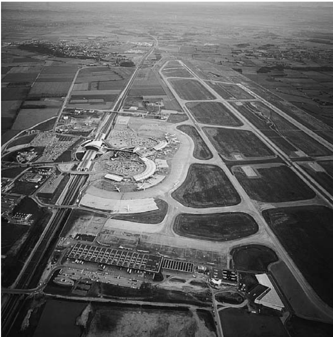
11.2 Linked terminals at Lyon-Satolas Airport, France. Architects: Curtelin Ricard Bergeret/Scott Brownrigg and Turner/Santiago Calatrava.
