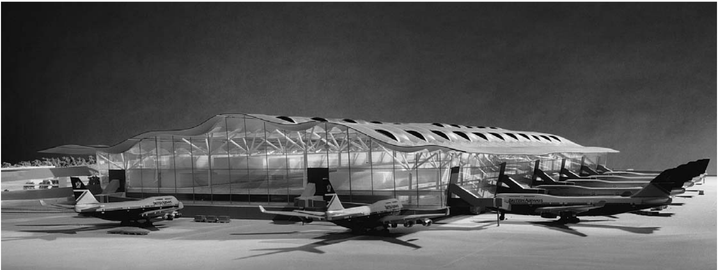
5.10 Reducing the visual impact of terminals by varying the roof profile and stepping at the edge helps to absorb large buildings into the open landscape of airports. Heathrow Terminal 5, UK. Original design by Richard Rogers Partnership.
