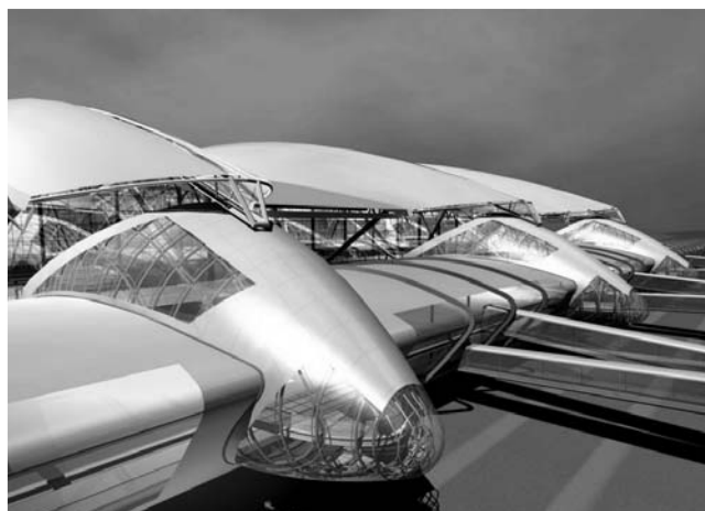
3.1 Modern airport terminals often ape the technology of the aircraft they serve. Xian Airport, China. Architect: Llewelyn Davies.
