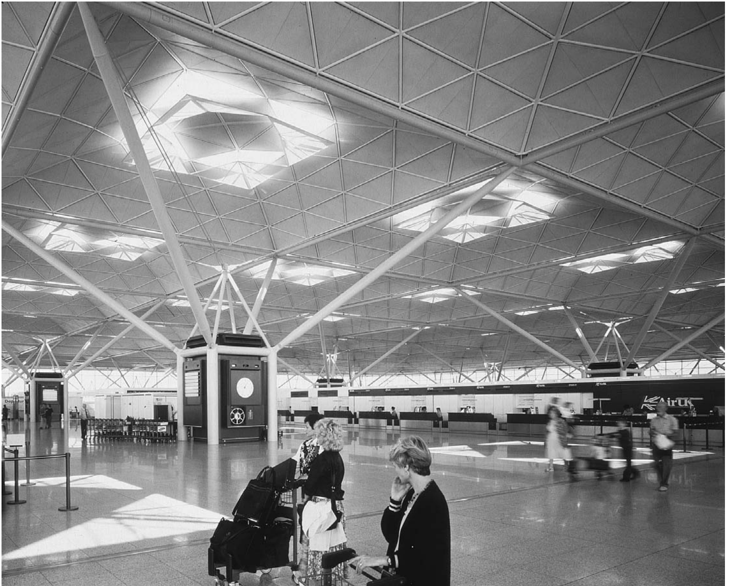
13.11 Daylight and artificial light need to define routes and important areas such as check-in desks. Stansted Airport, UK. Architects: Foster and Partners.
