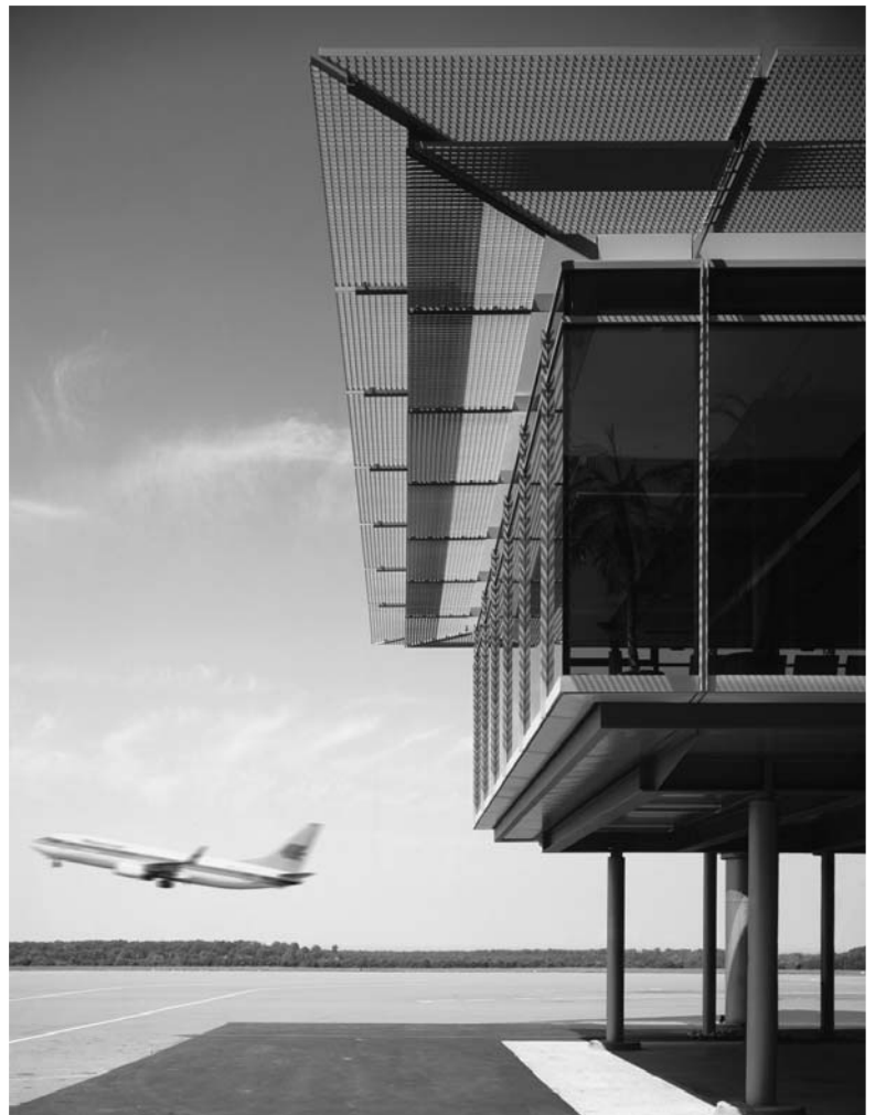
2.8 Tectonic construction is a feature of recent terminal design. Paderborn-Lippstadt Airport, Germany. Architects: Von Gerkan, Marg & Partner.
