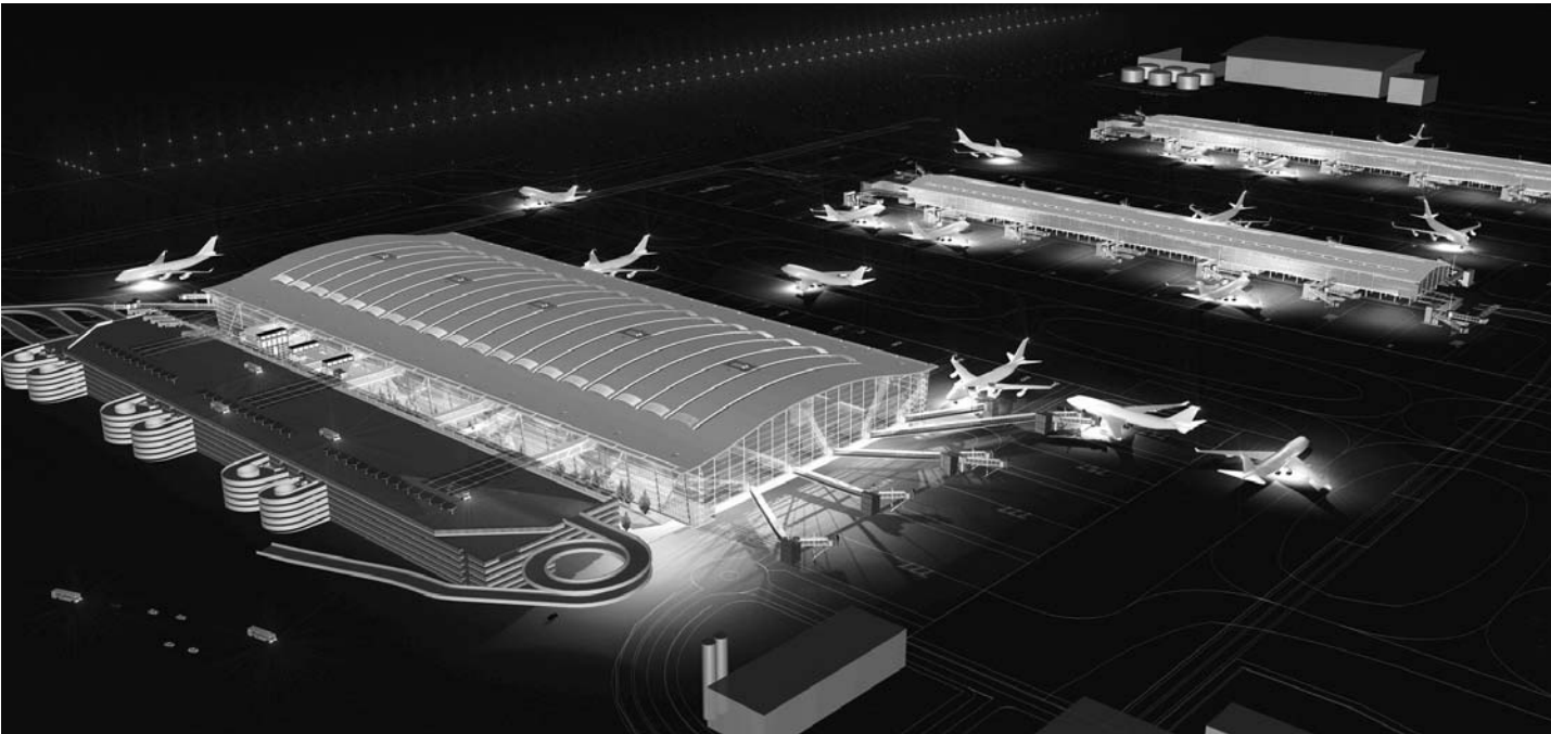
15.23 Aerial view of revised design for Terminal 5 at Heathrow. Architects: Richard Rogers Partnership.
