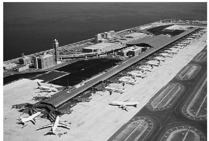
11.3 Linear gate pier linked to a central terminal at Kansai Airport, Osaka, Japan. Architects: Renzo Piano Building Workshop.
