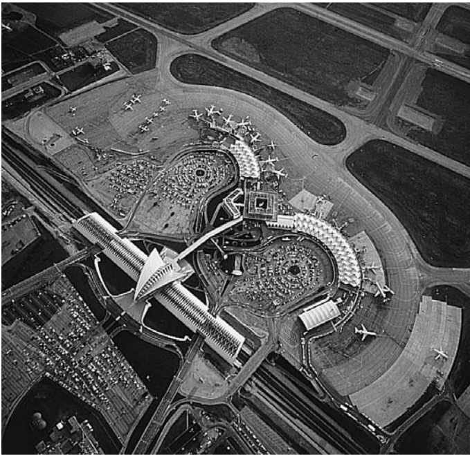
4.1 The classification of airports reflects passenger movements and architectural ambition. Lyon-Satolas Airport, France. Architects: Curtelin Ricard Bergeret/Scott Brownrigg and Turner/Santiago Calatrava.
