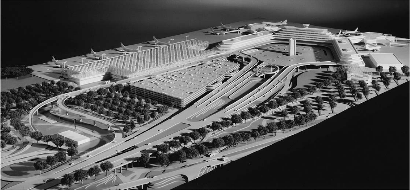
11.11 Airports increasingly support a variety of terminal designs. Here at Cologne/Bonn Airport, Germany, there are multilevel, unit and satellite terminals forming a harmonious composition. Architects: Murphy/Jahn.
