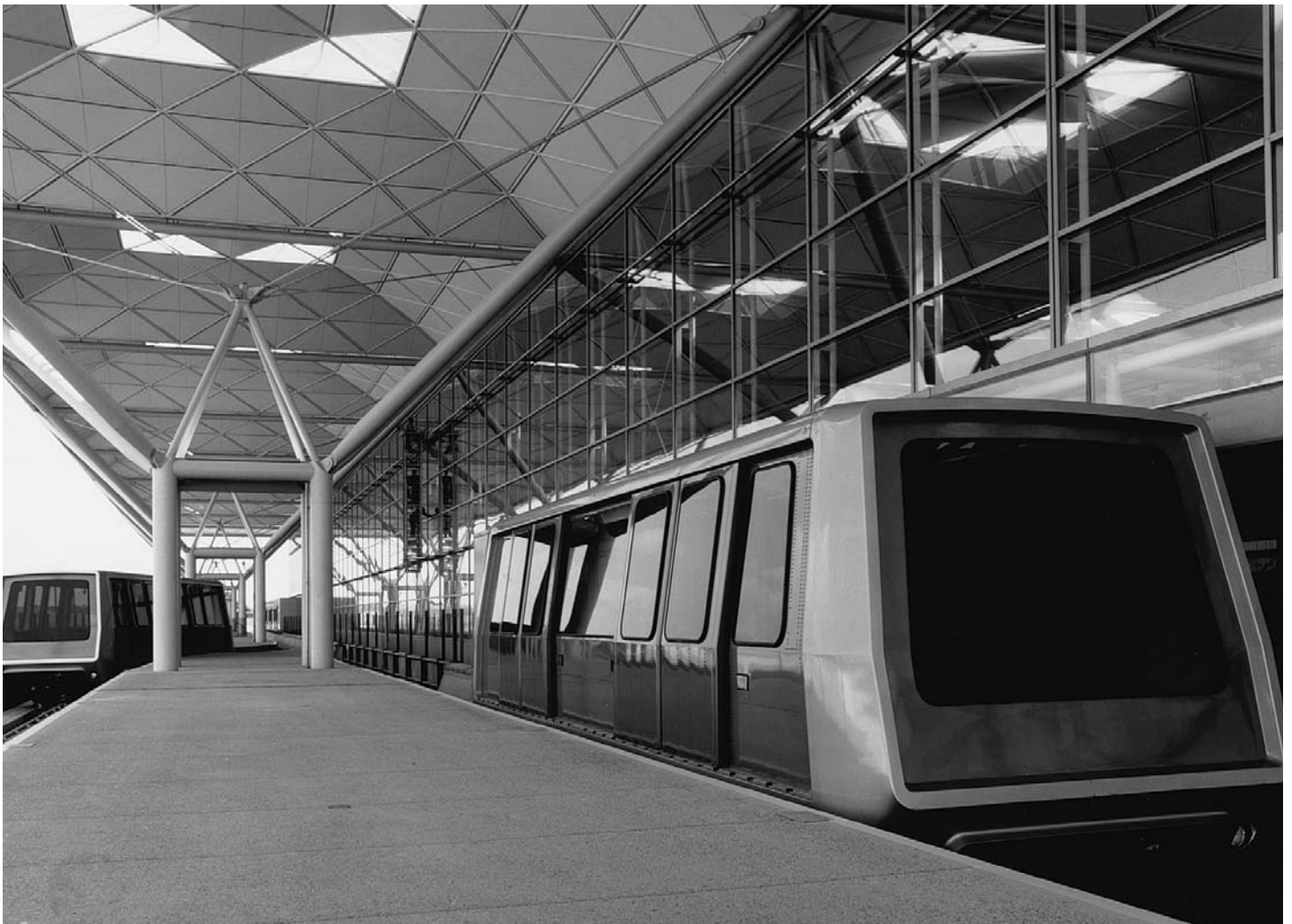
16.2 Light rail trams are used to transport passengers from the terminal to the satellites at Stansted Airport, UK. Each AEG Westinghouse tram cost £1 million. Architects: Foster and Partners.
