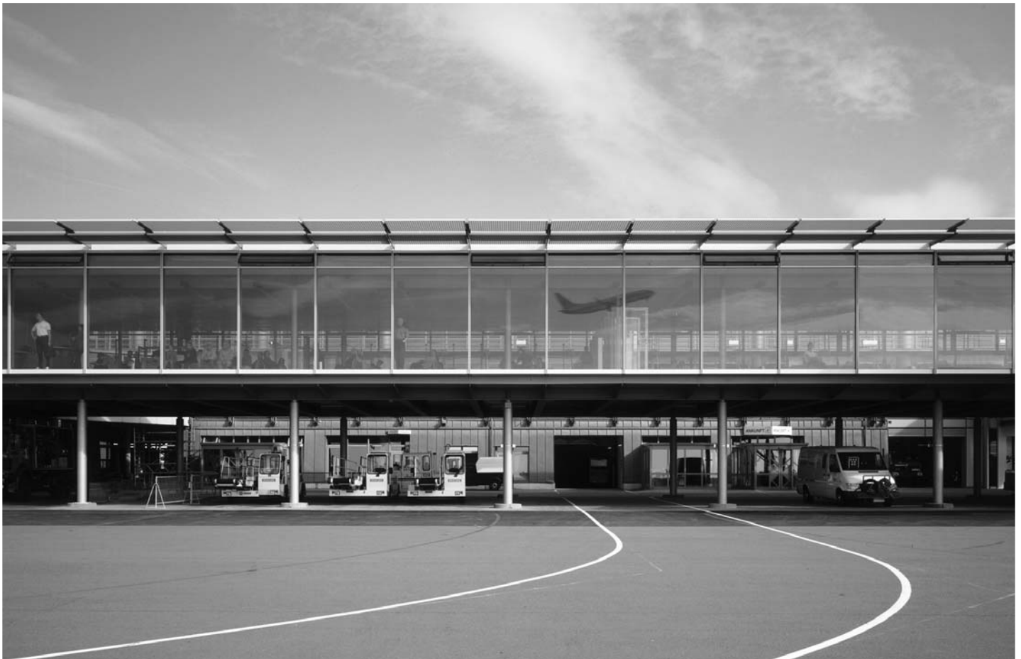
10.3 Airside view of passenger handling at rear of terminal. Paderborn-Lippstadt Airport, Germany. Architects: Von Gerkan, Marg & Partner.
