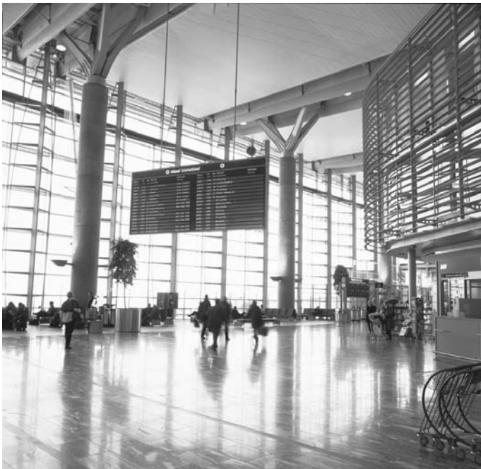
13.9 The structural system at Oslo Airport becomes lighter and more organic as the building rises.
