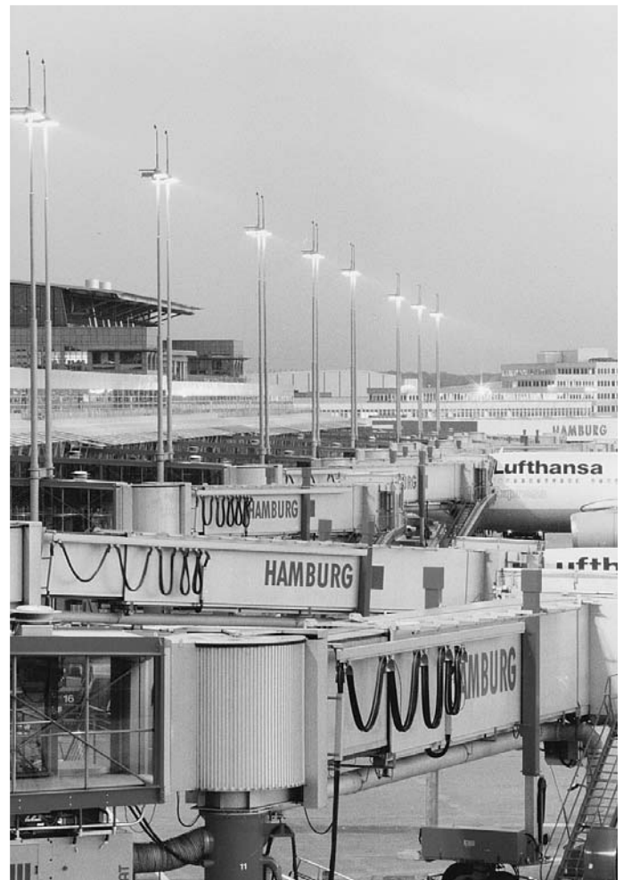
1.14 The design of aircraft and loading systems tends to determine airport and terminal layout. Hamburg Airport, Germany. Architects: Von Gerkan, Marg & Partner.
