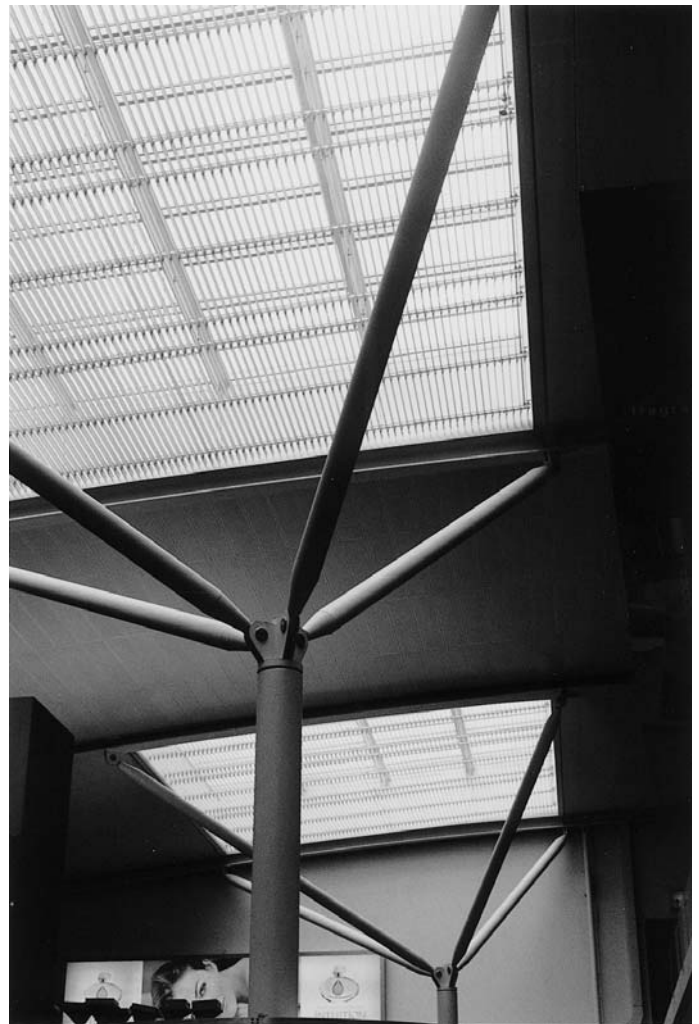
13.10 The integration of natural light and architectural structure increase the sense of weightlessness. Heathrow Terminal One Airside Link.
