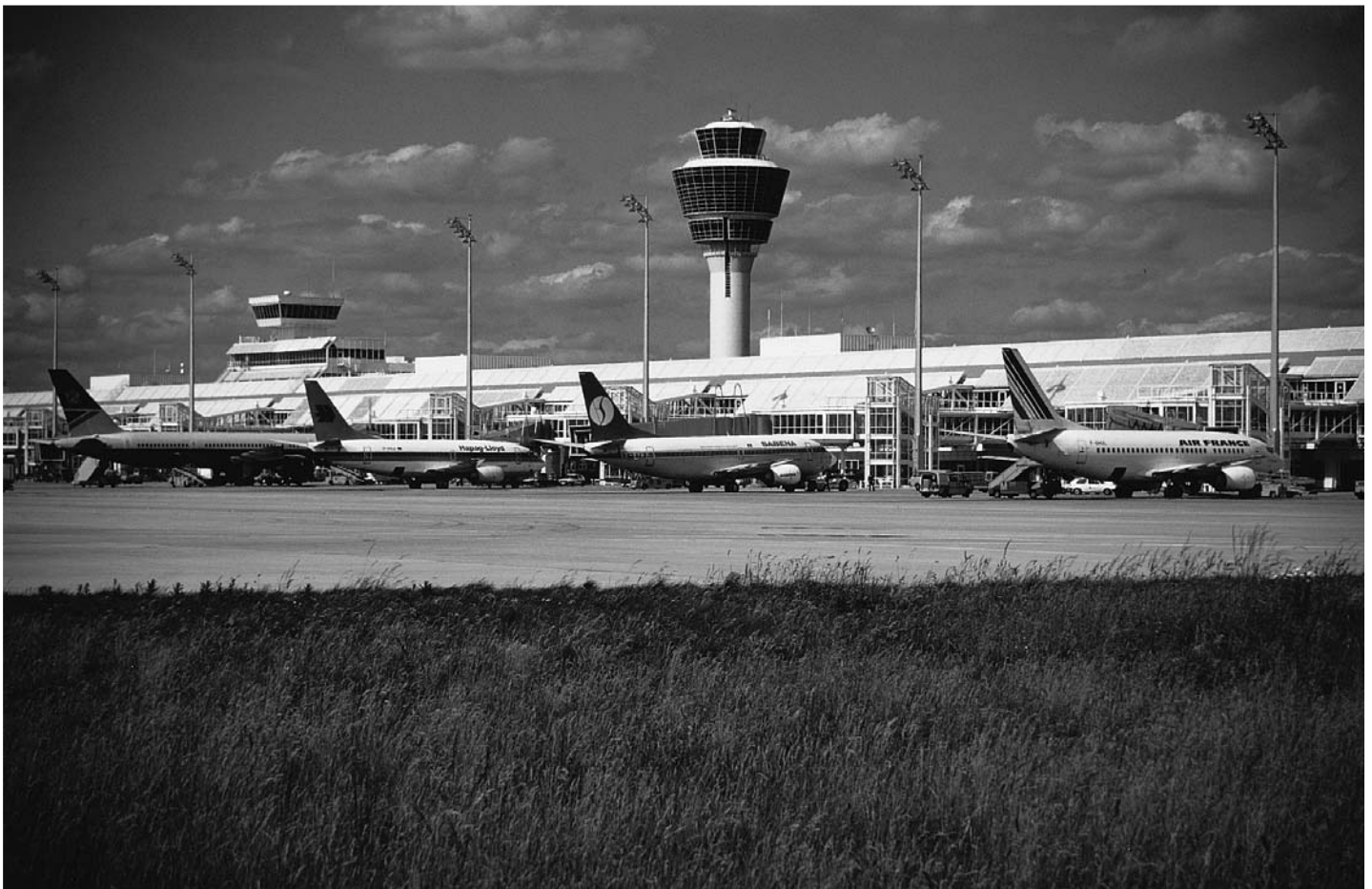
8.4 Changes in aircraft design trigger alterations to gate design. Munich Airport, Germany. Architects: Prof. von Busse, Blees, Kampmann & Buch.
