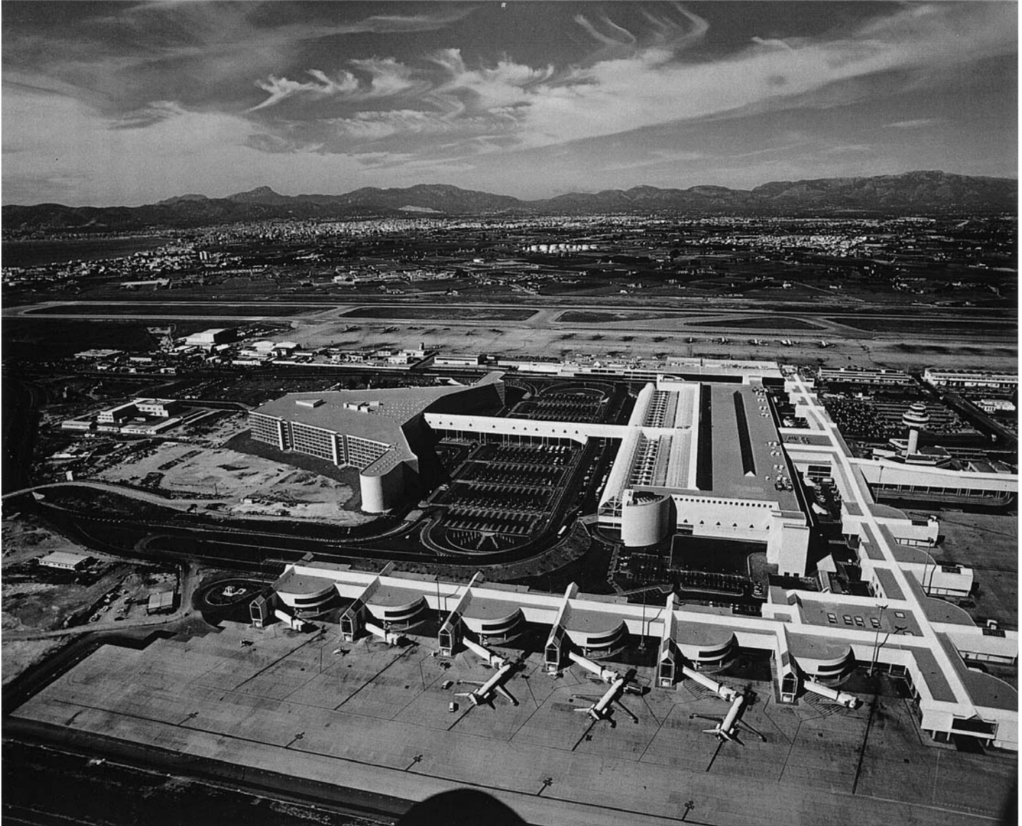
11.10 Palma Airport, Majorca, is a good example of a central terminal with gate piers parallel and at right angles to the main building. Notice the way gate lounges provide views over the apron.
