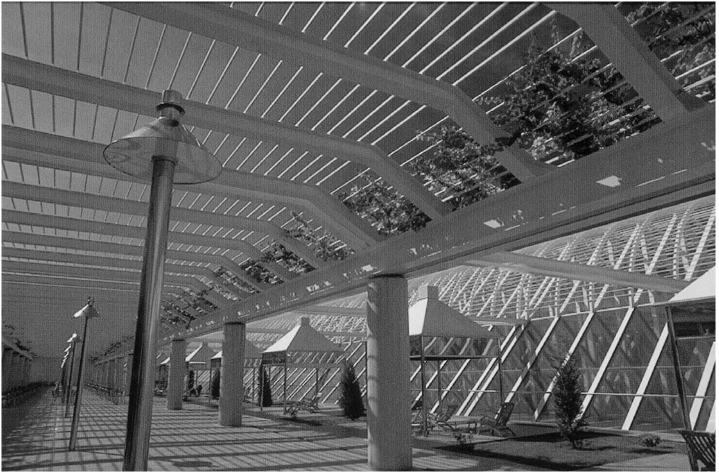
16.19 Sun-bathing terrace on roof of Palma Airport.
