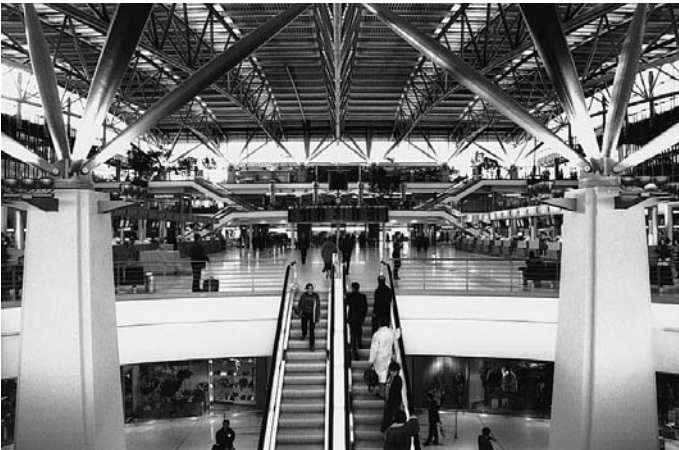
16.14 Hamburg Airport, Germany. Architects: Von Gerkan, Marg & Partner.
