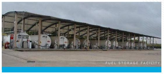
operations on their designated apron or facility. **Figure 1-6** depicts the current fuel tank setup and divisions based on lease with 95,000 gallons available for tenant lease as negotiated by the airport. Fuel resupply is accomplished via a secure/gated lane between the storage tanks and Addison Road entry of which is near Taxilane Quebec and exit is near Taxilane Papa.
