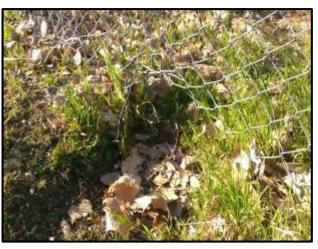
etc.) until a permanent fix can be made. Several gaps under the fence were observed on the western side of the security perimeter fence.
