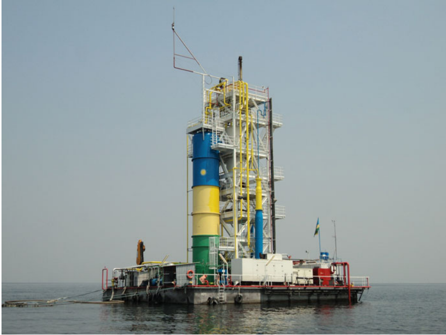
Fig. 1.4 Gas extraction facility of Kibuye Power 1 (KP1), the first pilot plant for large-scale commercial methane extraction from Lake Kivu that started operating in January 2009 (Photo provided by Kibuye Power Ltd.)
