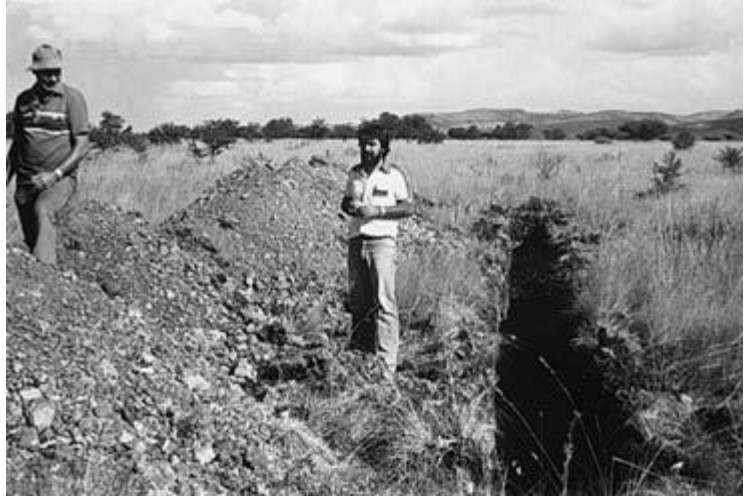
FIG. 5.8 Typical exploration trench, in this case on the South African Highveld.
