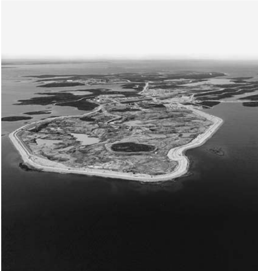
FIG. 17.21 Aerial view of pre-stripping of the A154 pipes at Diavik in 2002. (Courtesy Diavik Diamond Mines Inc.)
