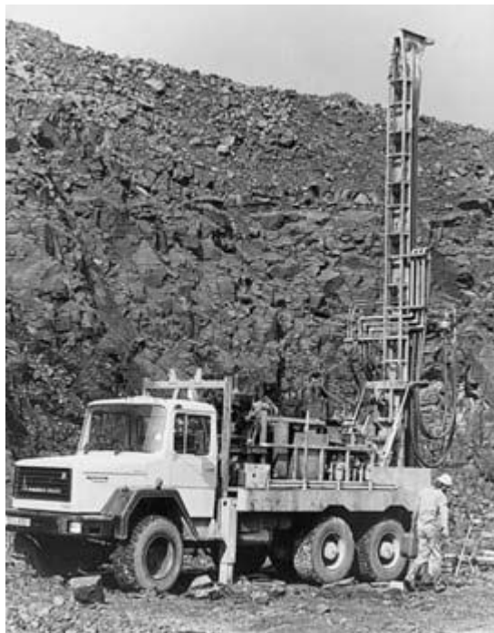
FIG. 12.3 A top-drive, multipurpose, flight auger drilling rig used to evaluate the resources on the Stud Farm property adjacent to Cliffe Hill Quarry.
