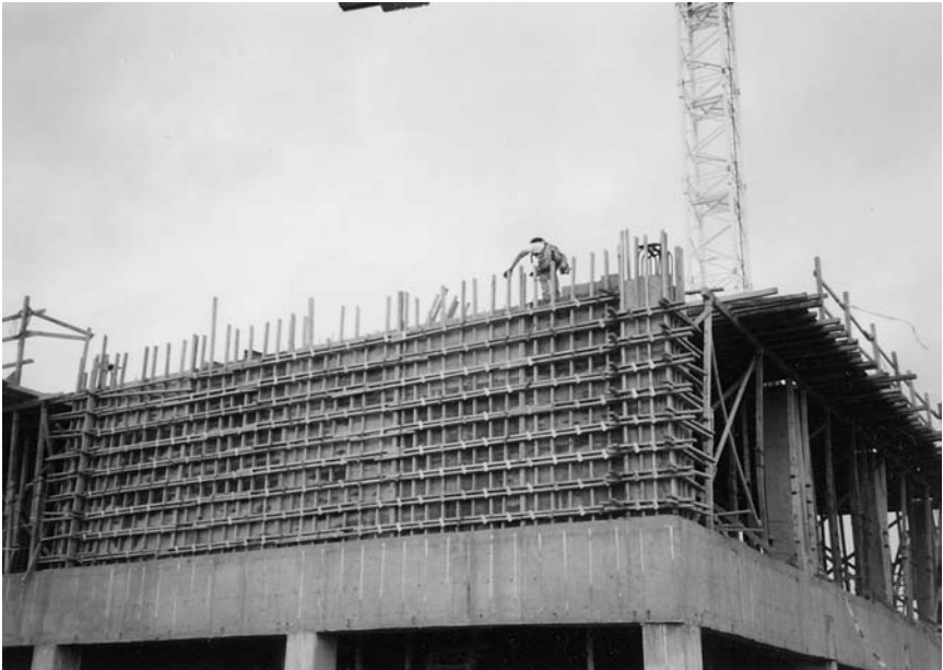
FIGURE 8.5 Plyform system for wall and column construction.
