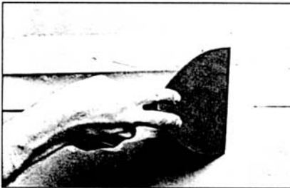
1. Fill Joint And Bed Tape Simultaneously
