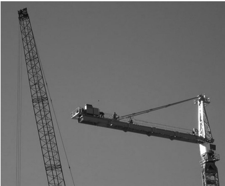
FIGURE 8.19 Positioning the counterdeck.
