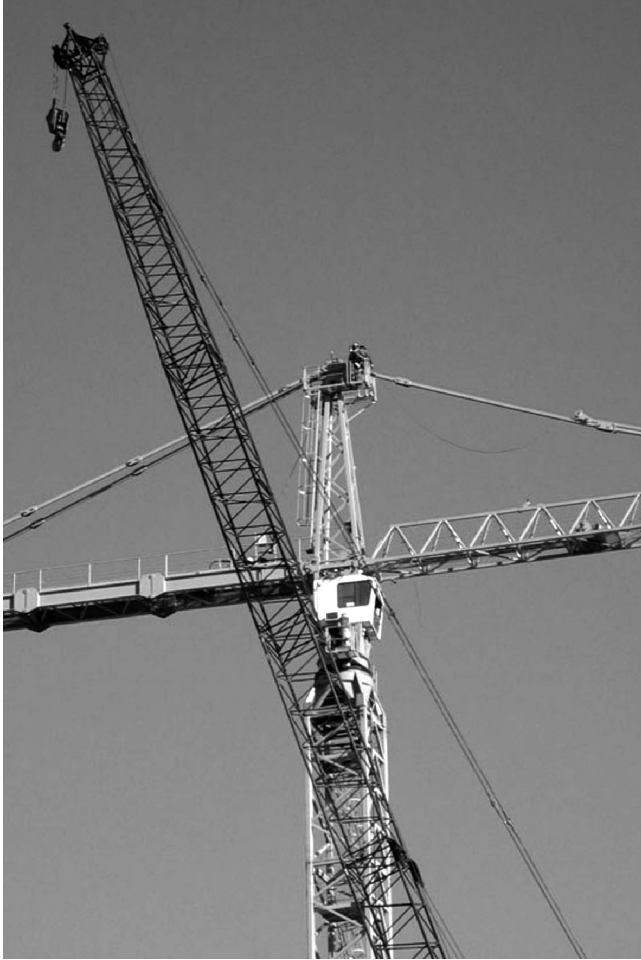
FIGURE 8.17 Riggers on the crane.
