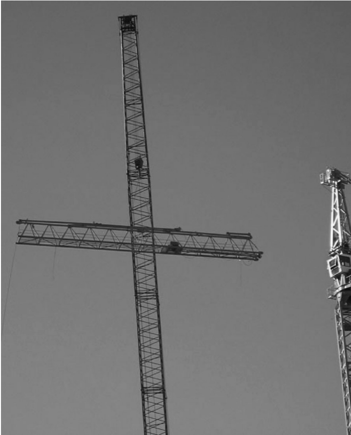
FIGURE 8.18 Disconnecting the remaining jib.
