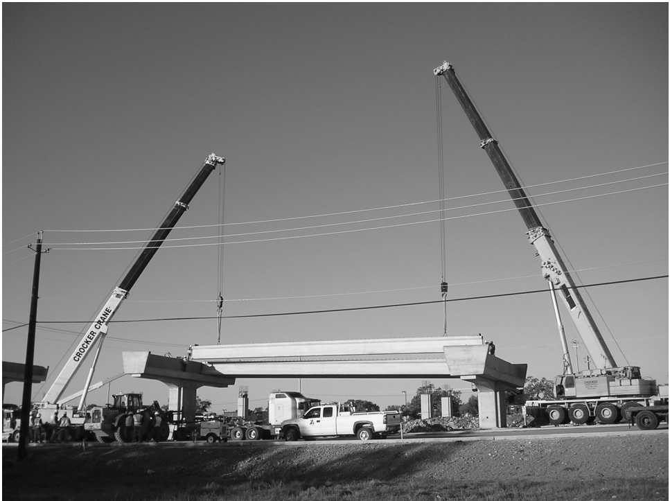
FIGURE 8.1 Dual lifting.
