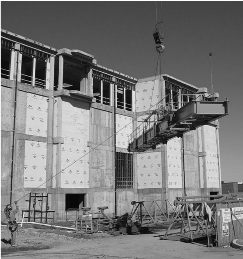
FIGURE 8.22 Lowering the counterdeck.
