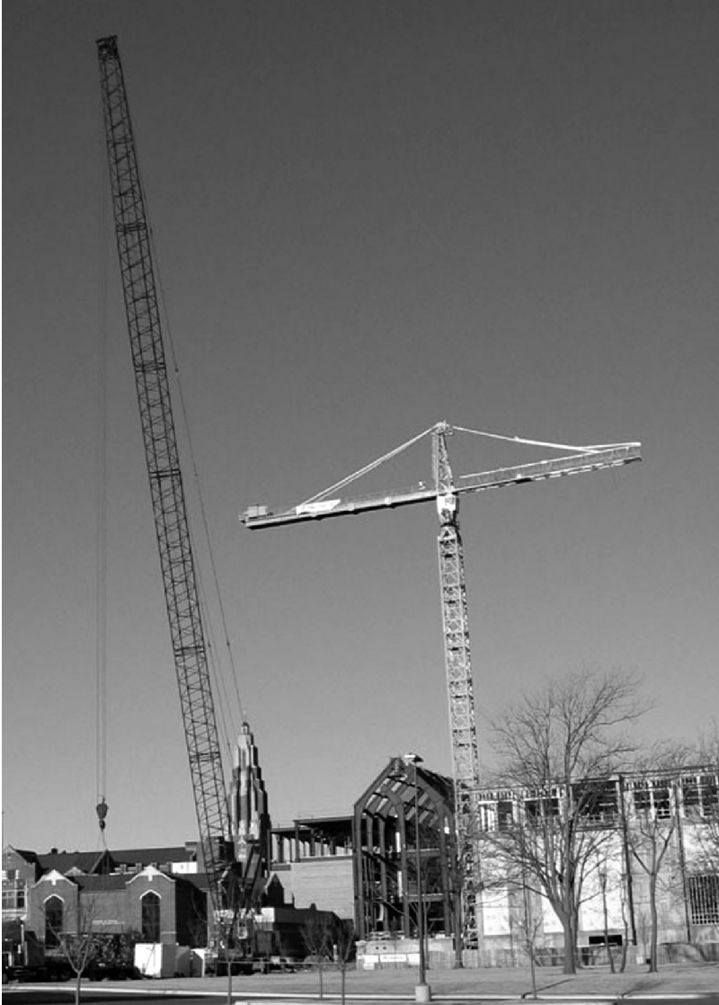
FIGURE 8.15 Two jib sections dismantled.
