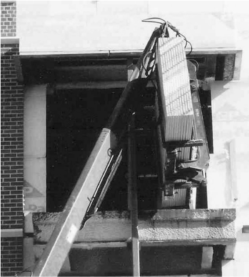
FIGURE 4.25 Sheetrock attachment.
