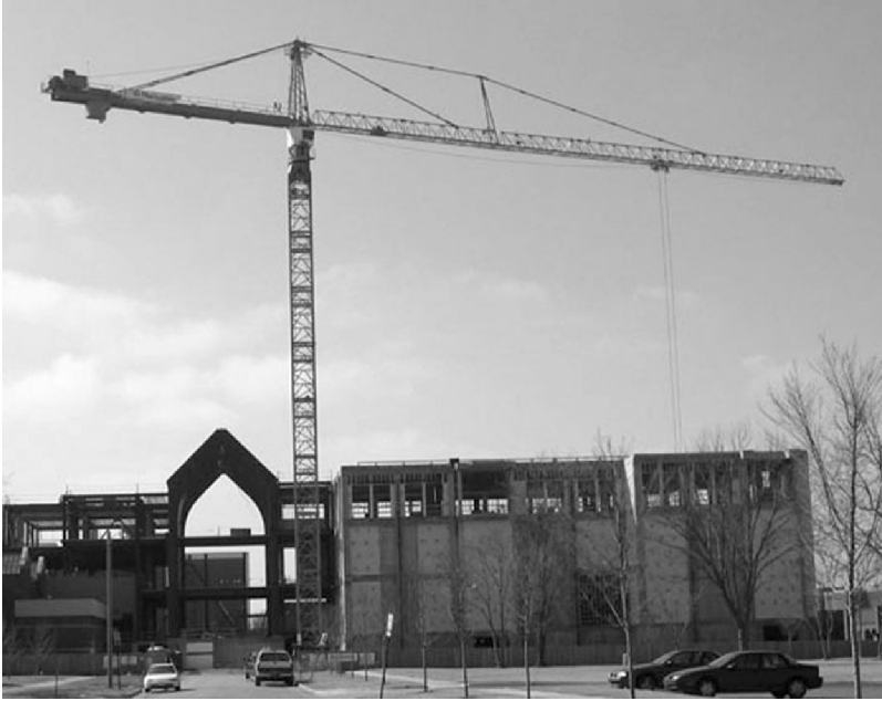
FIGURE 8.12 Horizontal jib tower crane.
