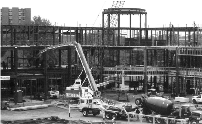
FIGURE 8.5 Pumping elevated flatwork.
