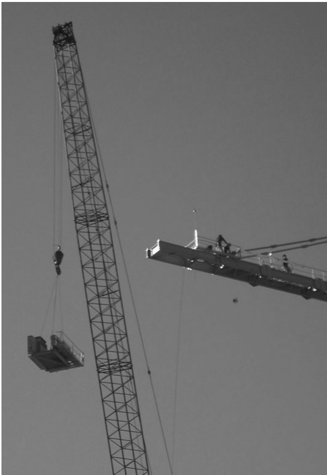
FIGURE 8.20 Removing the motor.
