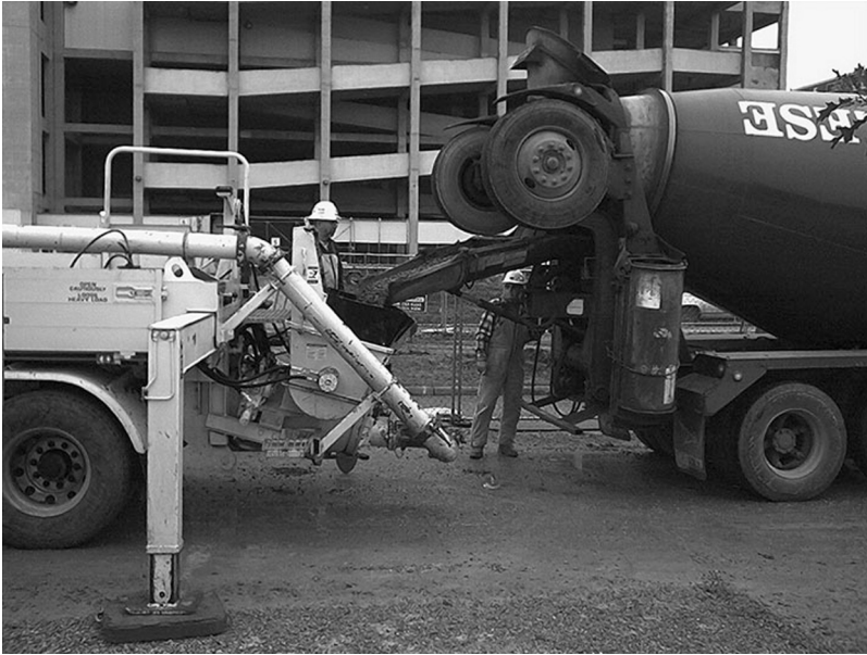
FIGURE 8.3 Chuting concrete into the pump hopper.
