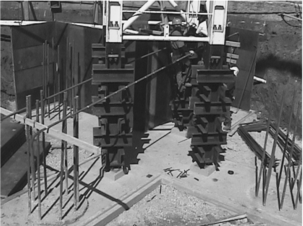
FIGURE 8.10 Tower base prior to pour.
