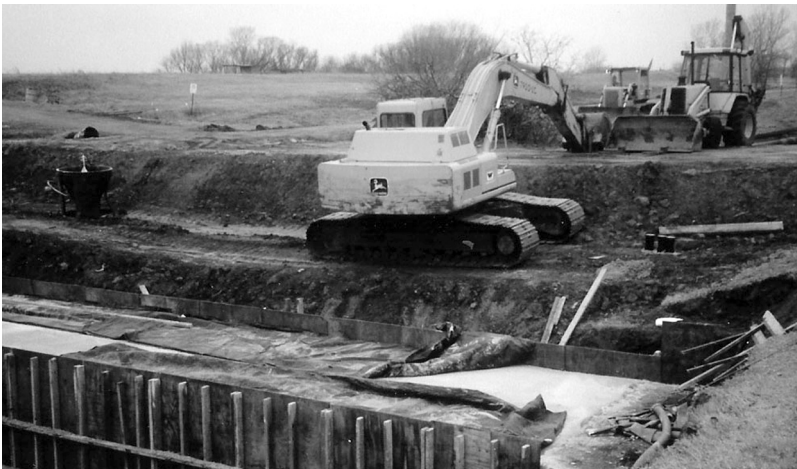
FIGURE 4.7 Excavator on a bench.
