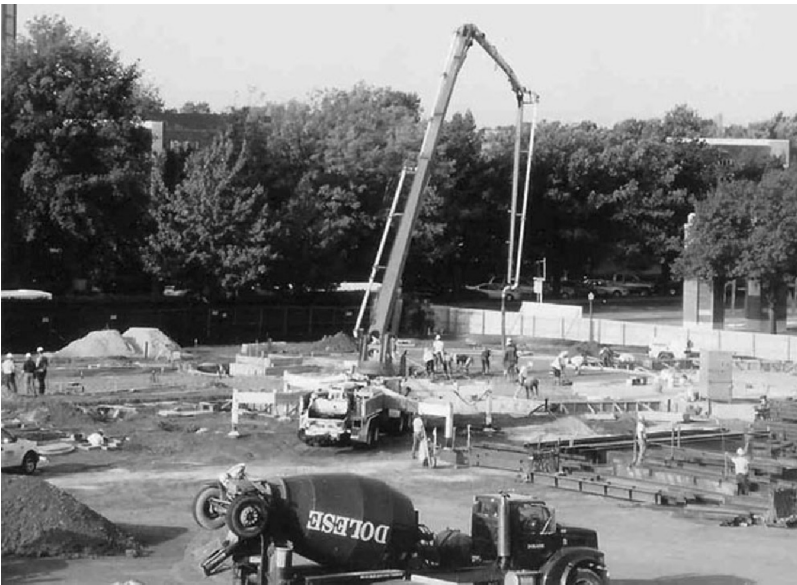
FIGURE 8.4 Pumping a slab on-grade.
