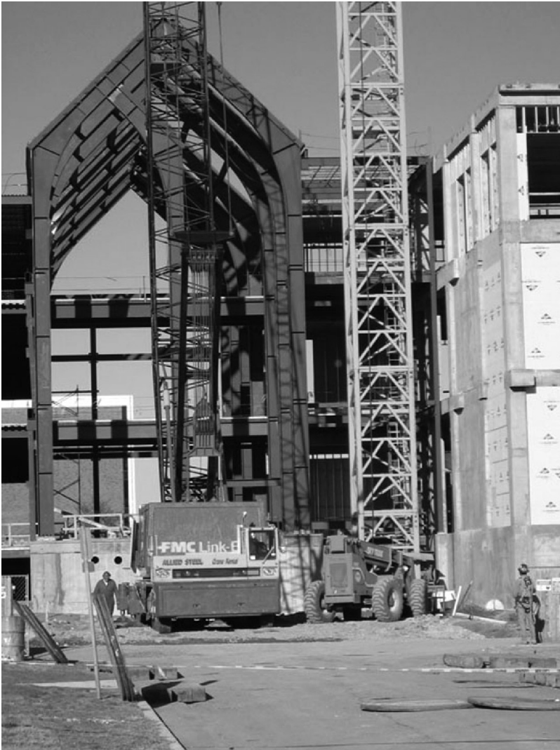
FIGURE 8.16 Support crane move.
