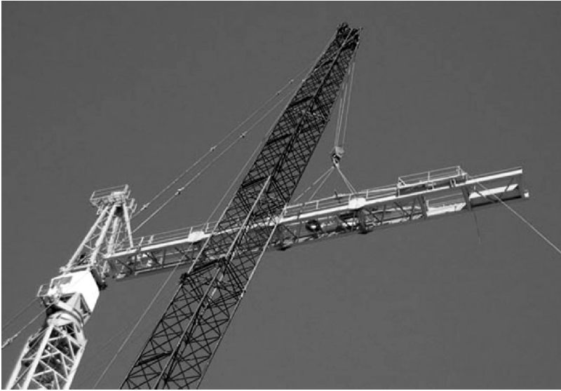
FIGURE 8.21 Dismantling the counterdeck.
